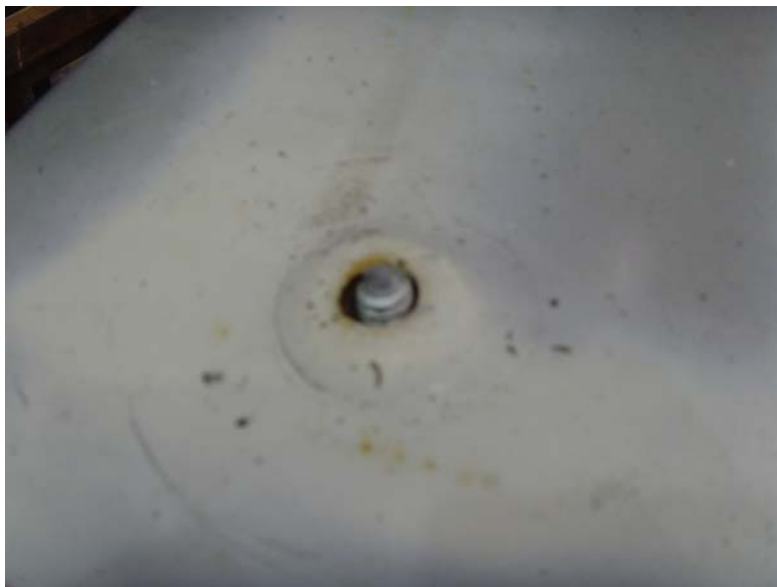
Plate 6 Failure of Lifting Eye
