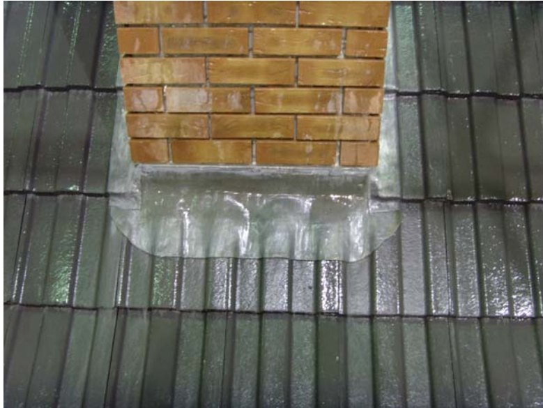
Plate 11 Detailing for Mono-pitch Chimney
