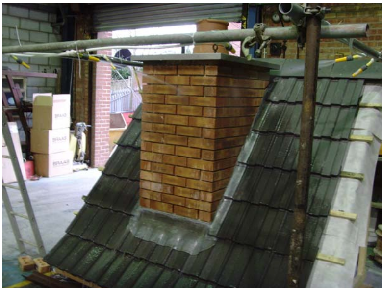
Plate 10 Mon-pitch Chimney under Water Tightness Testing
